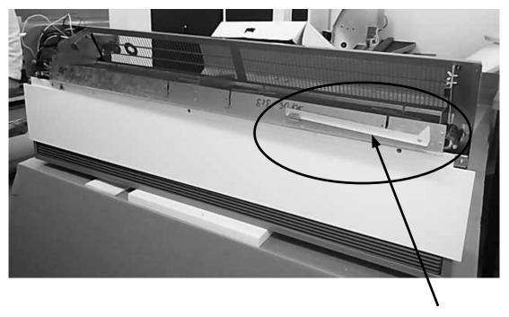
When the coil is detached, the pop rivet holding the front hatch locking device shall be drilled out and be refitted on the new coil with a new pop rivet.
