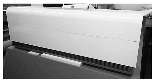
Detach the front plate by removing the allen key screws.
